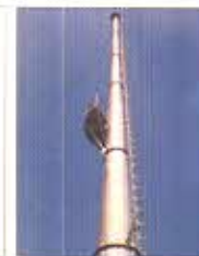
Self Supported Chimney
