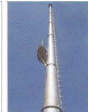
Self Supported Chimney
