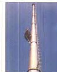
Self Supported Chimney
